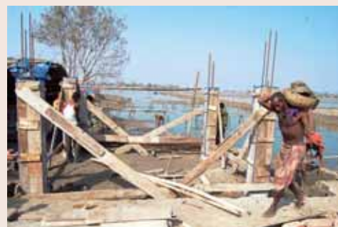
Image 1: Community participation in building disaster resilient houses (Source: Kabir, 2017).
